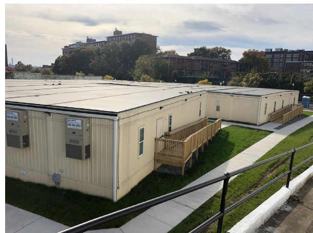
Photo above of prefabricated modular classrooms manufactured by Wilmot Modular, Inc. ( https://www.wilmotmodular.com/blog/how-to-get-your-portable-classroom-in-time-for-the-new-school-year )
