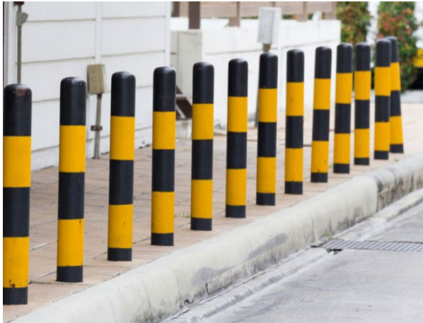
Above photo of typical bollards used for separation and barriers between vehicles and pedestrians.
